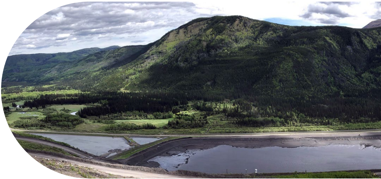
Wolverine Mine's tailings storage facility
