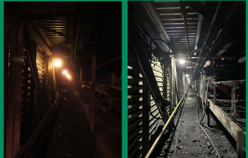
Image: Before (left) and after (right) photos of energy efficient lighting upgrades at Quintette
